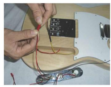
Connect the cables of the pickups to the cables which are on the switch.
